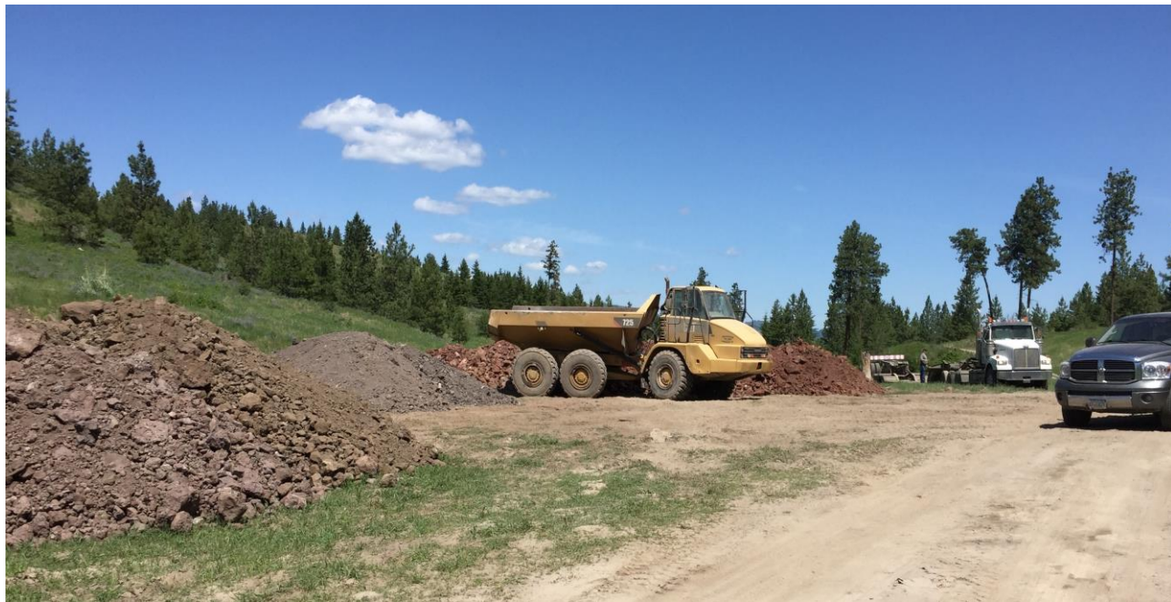
Stockpiling TransCanada Ore at Plant Site
